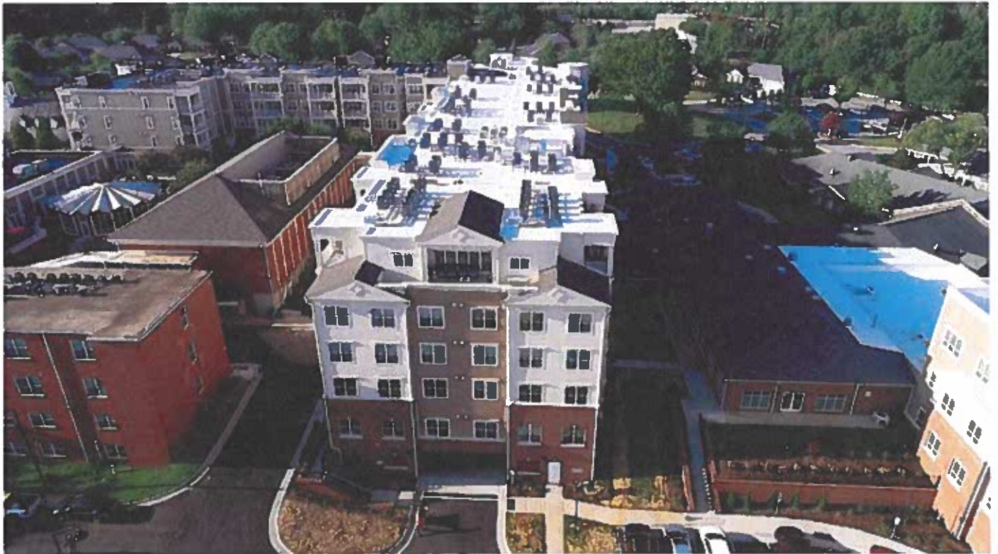
Independent Living – North Elevation – Garage entrance
