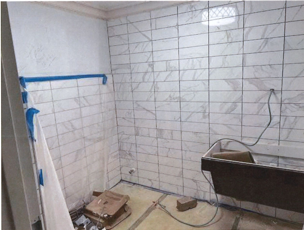
AL/MC – Public Restroom Lower Level
